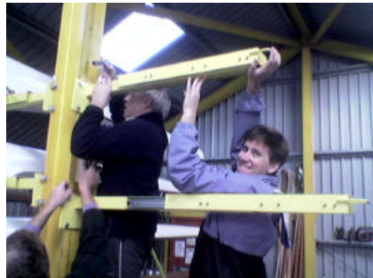
Andrew and Mark at work on the racking
